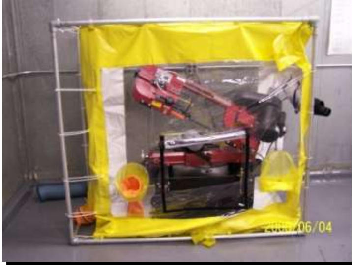
Band Saw Containment Tent
